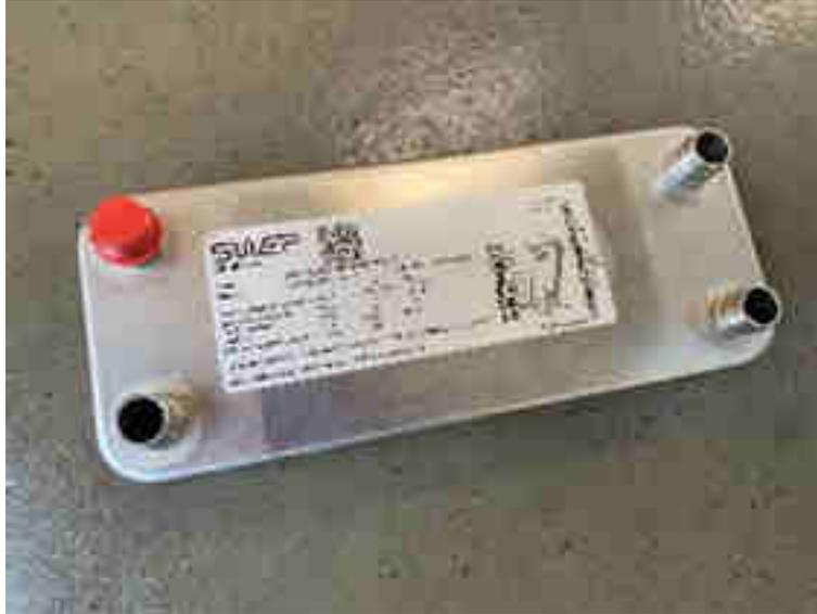
Figure 88: Coolant-coolant heat exchanger for QUIET thermal management system set-up
